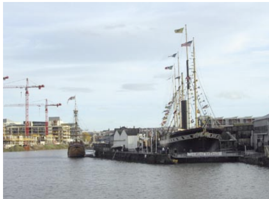
Gas Ferry Road Bristol BS1 6TY
